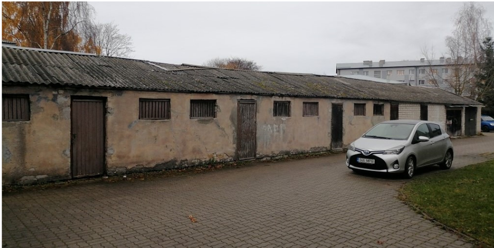
Vaade loodest (Foto: ApexAB november 2022)
