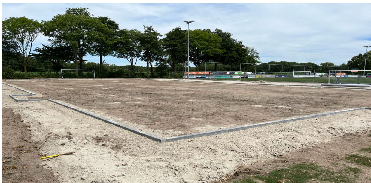
Figure 8 – example of crushed stone base construction
