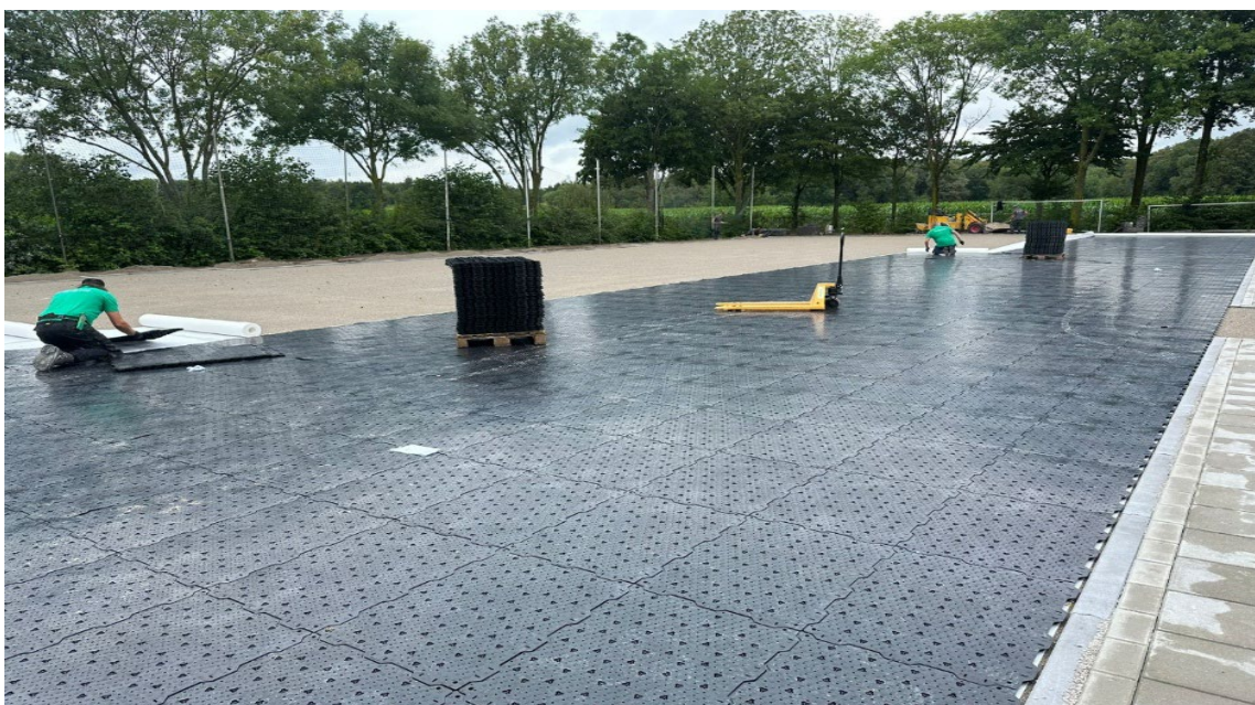
Figure 5 - installation of modular base panels
