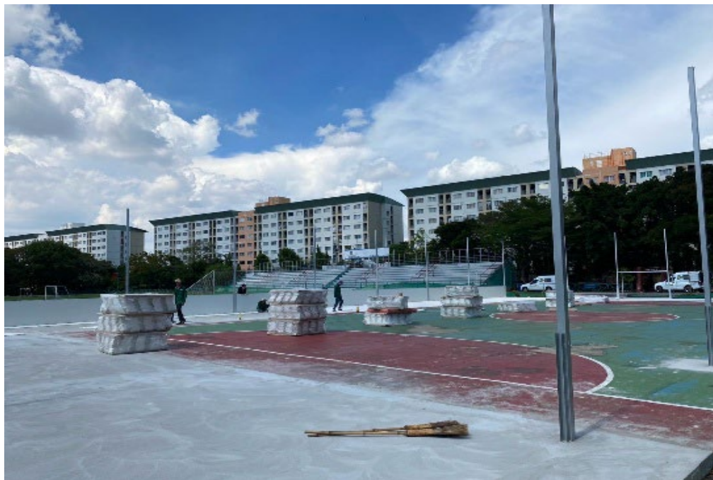
Figure 4 - conversion of existing paved area
